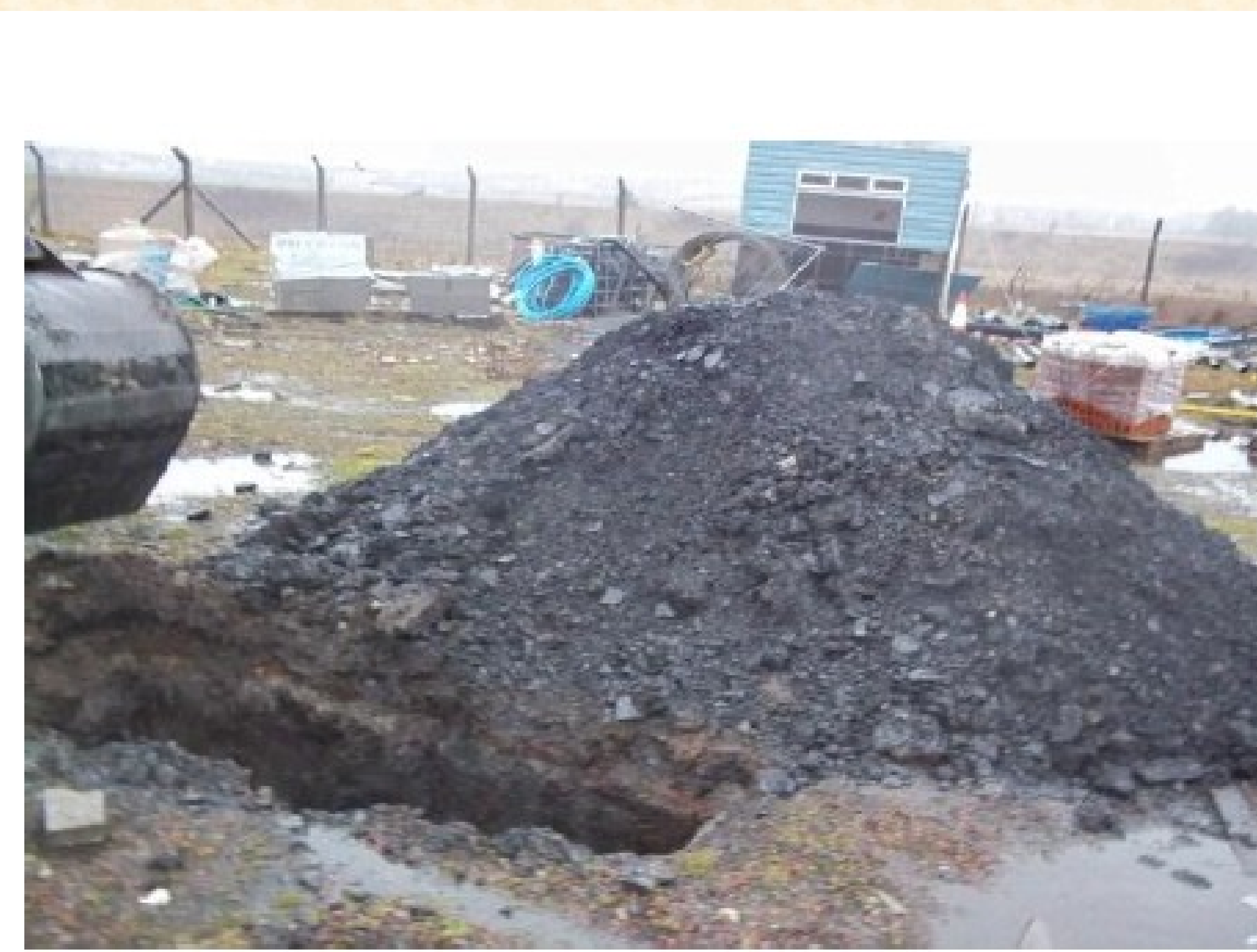
Figure 1 Hydrocarbon polluted soil removed from an underground tank being prepared for bioremediation treatment (URL1)
